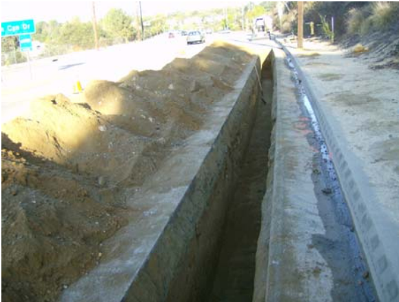
Trench Ready for Pipe Installation
