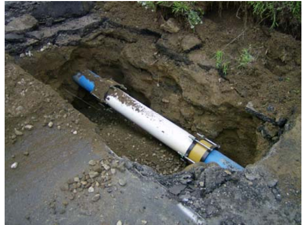
Pasadena Glen Water Main Repair Section
