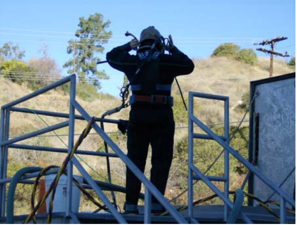
Wilcox Reservoir Inspection and Cleanout
