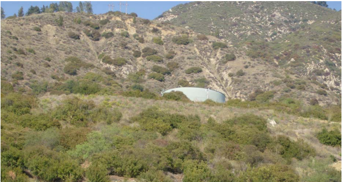
West Tank As Seen From Kinclair Drive
