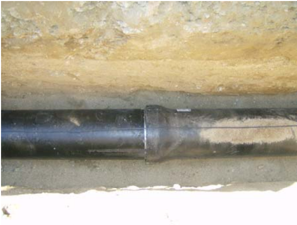
Ten Inch Ductile Iron Pipe
