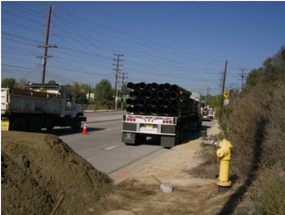
Pipe Delivery to Site
