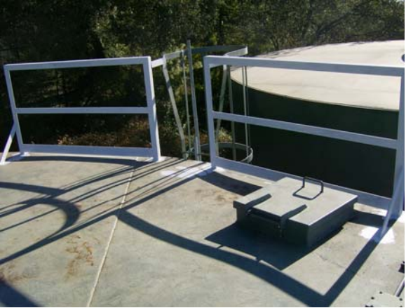
Holly Tanks Roof Safety Railings Installed
