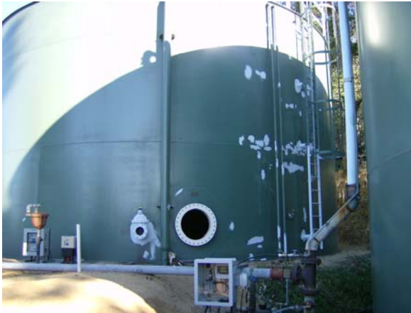
Holly Tanks Painting and Safety Upgrades
