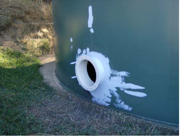
Refurbished Entry Hatches for Holly Tanks
